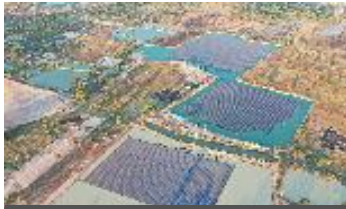
Floating Solar PV, TSB Co., Ltd., Thailand
