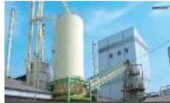
Biomass Co-Generation System, Fuji-Foods Corporation, Thailand
